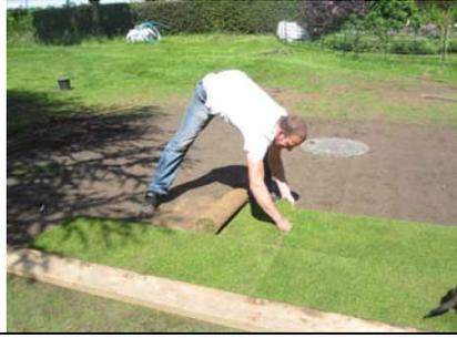
There was a well-advised wait of a couple of weeks and some rain to permit the covering to subside and settle before levelling off and turfing over. The turrets and manhole covers of the F-Line tank adjust for height and for level; adjustment continued even after the turf was down.
